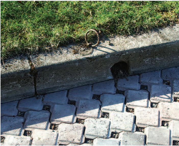
Figure 3. Portland has been reducing flows to combined sewer systems by disconnecting downspouts that daylight to street outlets like the one shown here. PICP offers another way to reduce combined sewer flows. The metal ring in the curb was a regional tradition that facilitates horse parking.
