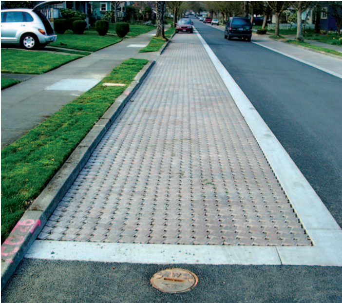
Figure 12. Capped, 4 ft (1.2 m) deep, 6 in. (150 mm) diameter perforated pipes serve as wells to monitor infiltration rates.
