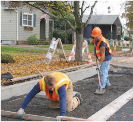
Figure 9. A makeshift screed levels the bedding course for the permeable pavers.
