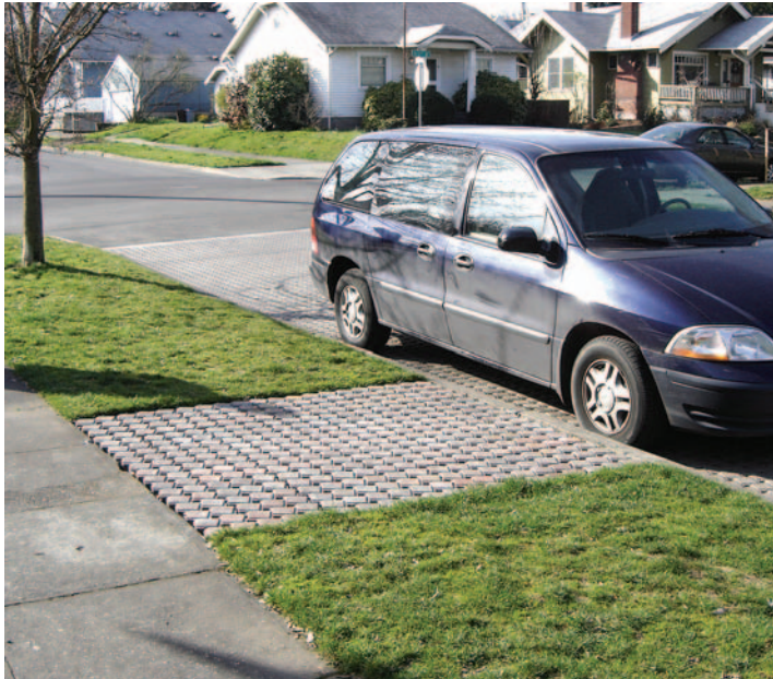
Neighborhood participation: a do-it-yourself resident replaced his front walk with spare pavers and bedding material.
