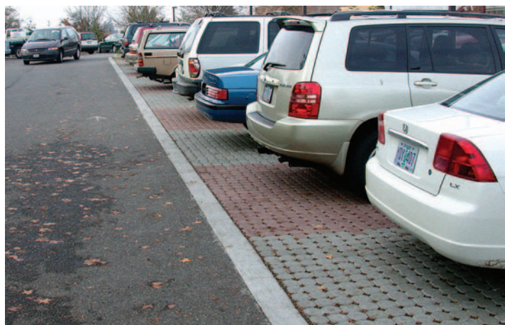
Figure 1. The City of Portland is not new to permeable pavements. The Multnomah Arts Center parking lot was one of the early projects.
