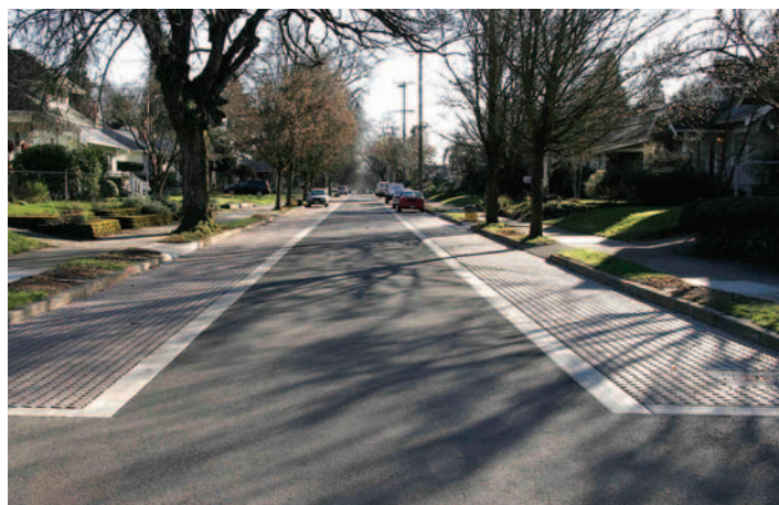
Figure 2. The permeable pavers receive runoff into an open-grade aggregate base, or "drainage blanket," that extends under the asphalt across the entire street. This boosts water storage and infiltration capacity.
