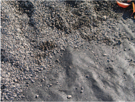
Figure 6. The bedding material was an Oregon DOT standard for small size, open graded stone.
